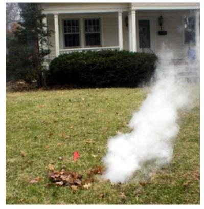
If you are outside and see smoke coming from a vent stack on a house, don't worry. The house is not on fire. This is normal. However, smoke coming from holes in the ground is not normal and is considered a defect. Town staff will photograph and log all defects like this. We will also contact property owners if a defect is found on private property.
